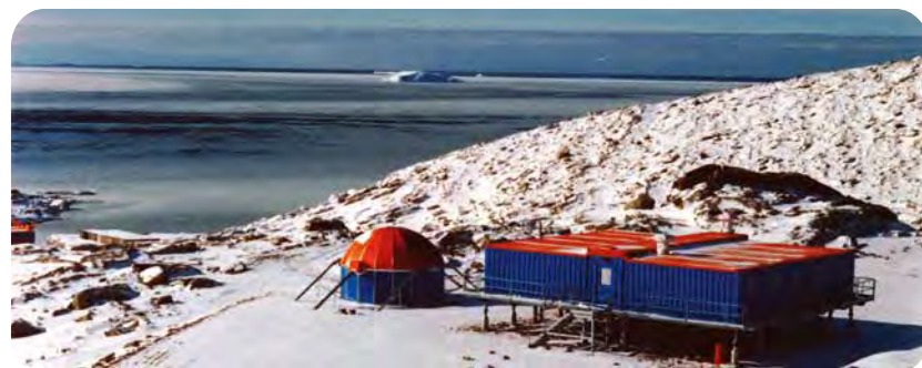
Kitchens and laundry facilities in the prefabricated units at the South Pole
